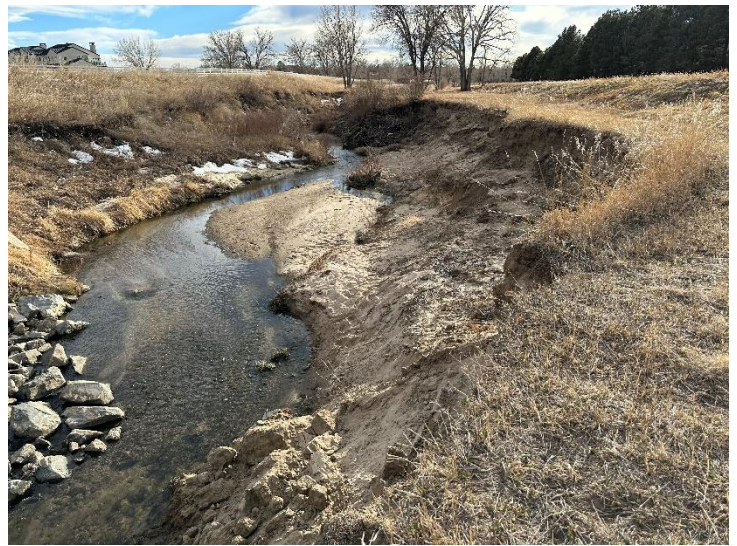
Figure 2: Looking Downstream at Pedestrian Crossing (2024)
