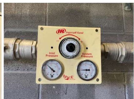
Reset pressure to 55 psi
