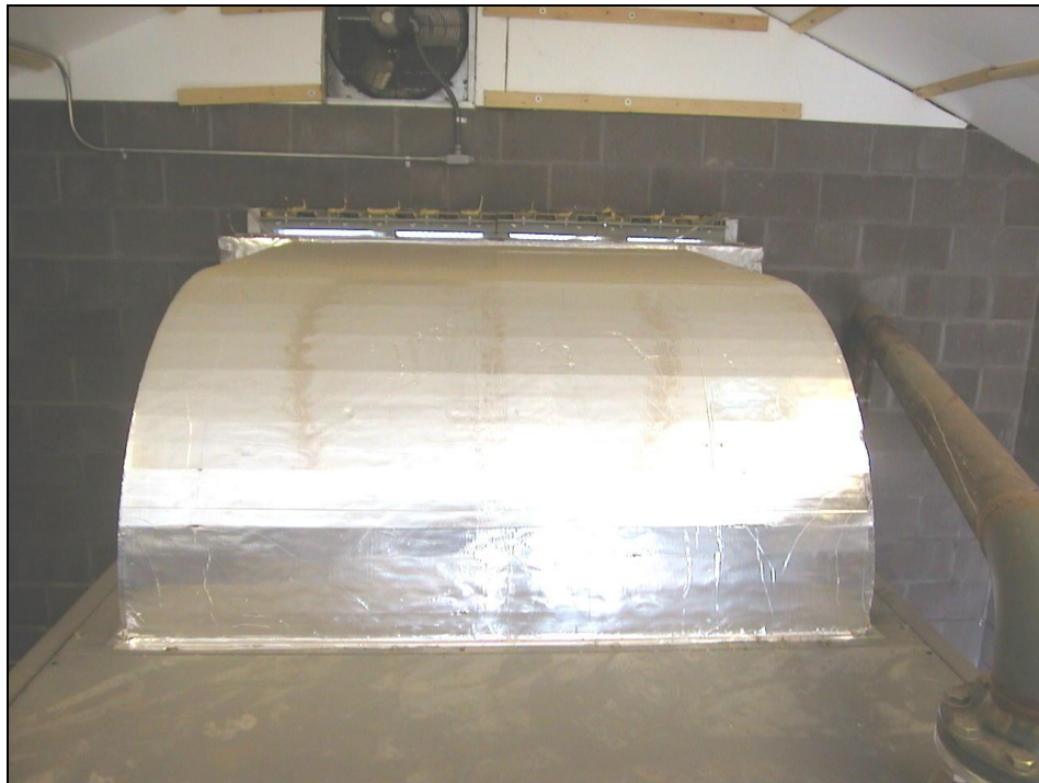
DISCHARGE DUCT INSULATION
