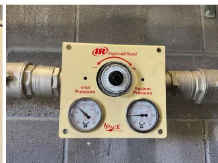
Reset pressure to 55 psi
