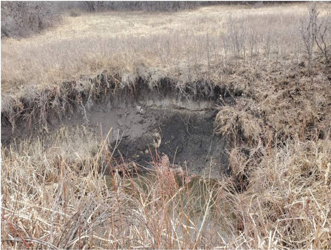
Photo of Bank Erosion on McMurdo Gulch Priority 3 Project (Courtesy of Muller Engineering)
